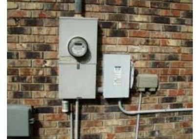
MAIN PANEL POWER SIZE: 200 amp +/- . The ampacity of the main service panel is adequate for the structure as it is presently being used.
