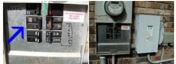
Note: The exterior panel has been equipped with a generator transfer outlet. If needed have the seller or an electrician give you directions on how to use this feature or how to complete this feature.
