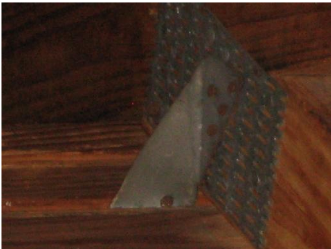
Roof to Wall Attachment - Clips
