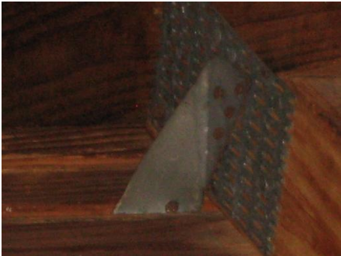
Roof to Wall Attachment - Clips
